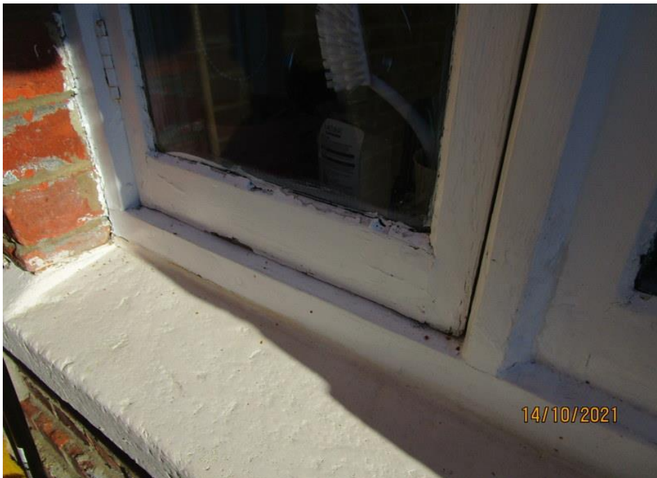
Deterioration affecting joinery and putty seals.
