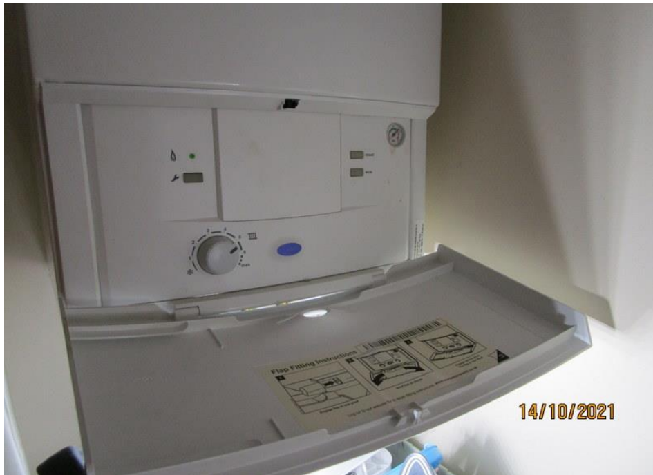
The central heating boiler is of a condensing type fitted in 2013.
