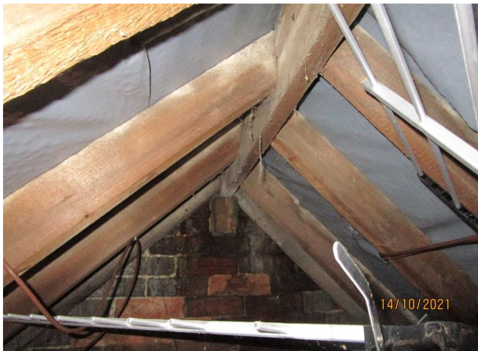
Roof structure showing rafters and purlin timber.
