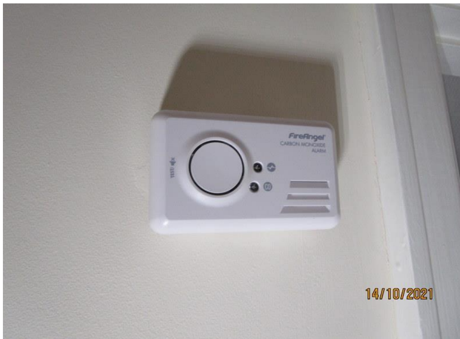
Carbon monoxide alarm.
