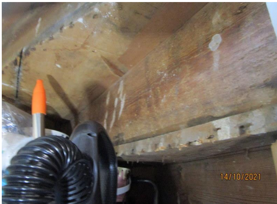
Stair joinery viewed from beneath.
