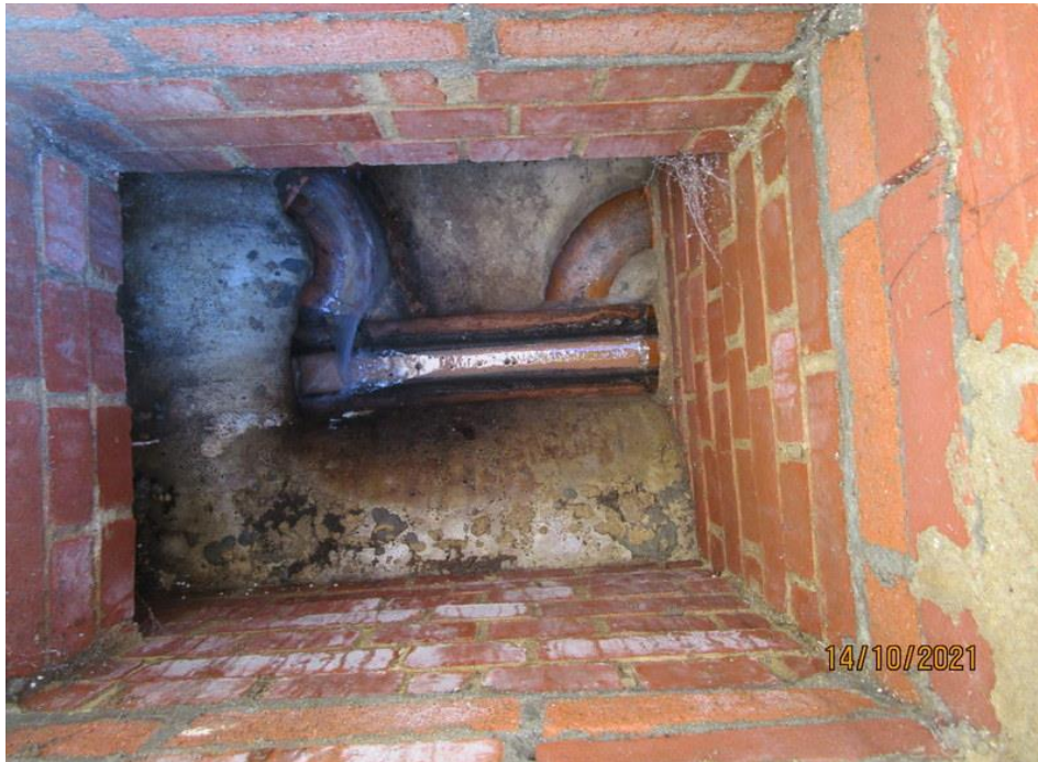
Clay drainage pipes to the rear of the property.
