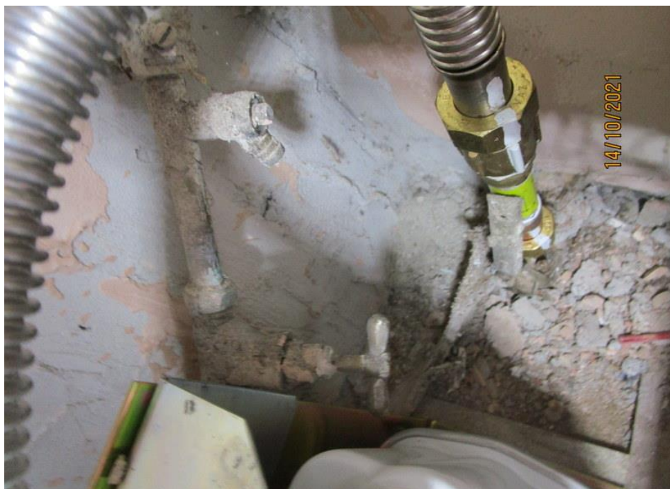
Gas pipes and water stop-tap.
