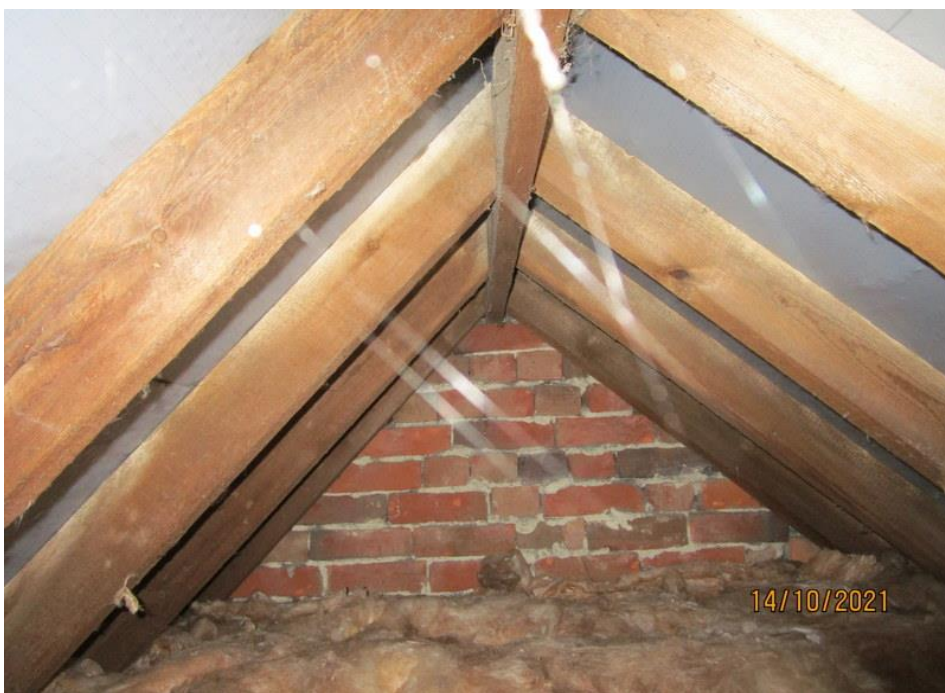
Brickwork to the side party wall showing again roof timbers.
