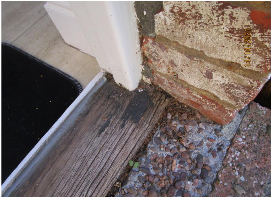
Deterioration affecting the rear door sill.
