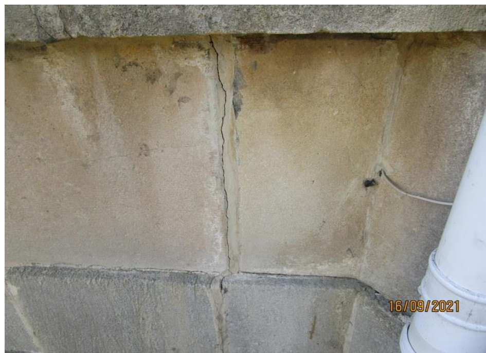
Cracks to the stonework around the front bay have been recently repaired but have reopened slightly.
