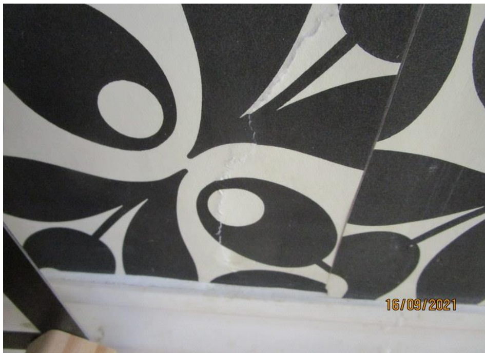
Evidence of cracking to the walls beneath plaster and paper finishes.
