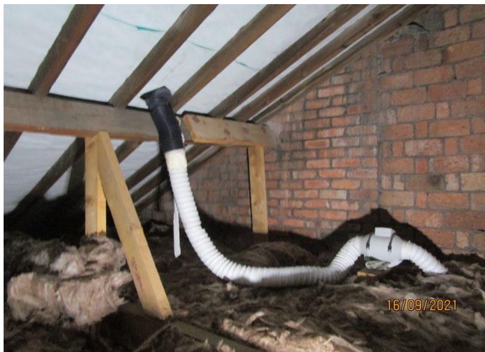
The rear part of the roof has been strengthened with the installation of extra struts and the purlin bearing has been improved.
