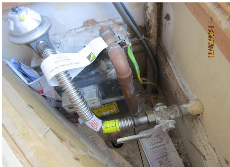
Gas meter showing electrical earth connection.
