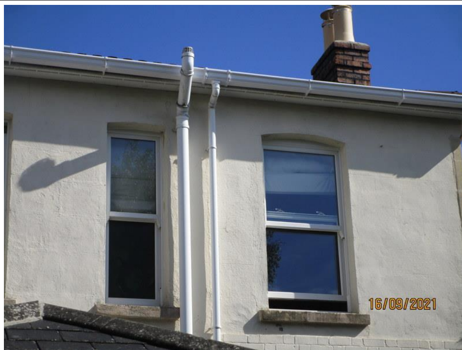
Rainwater fittings and render finishes to the upper rear wall.
