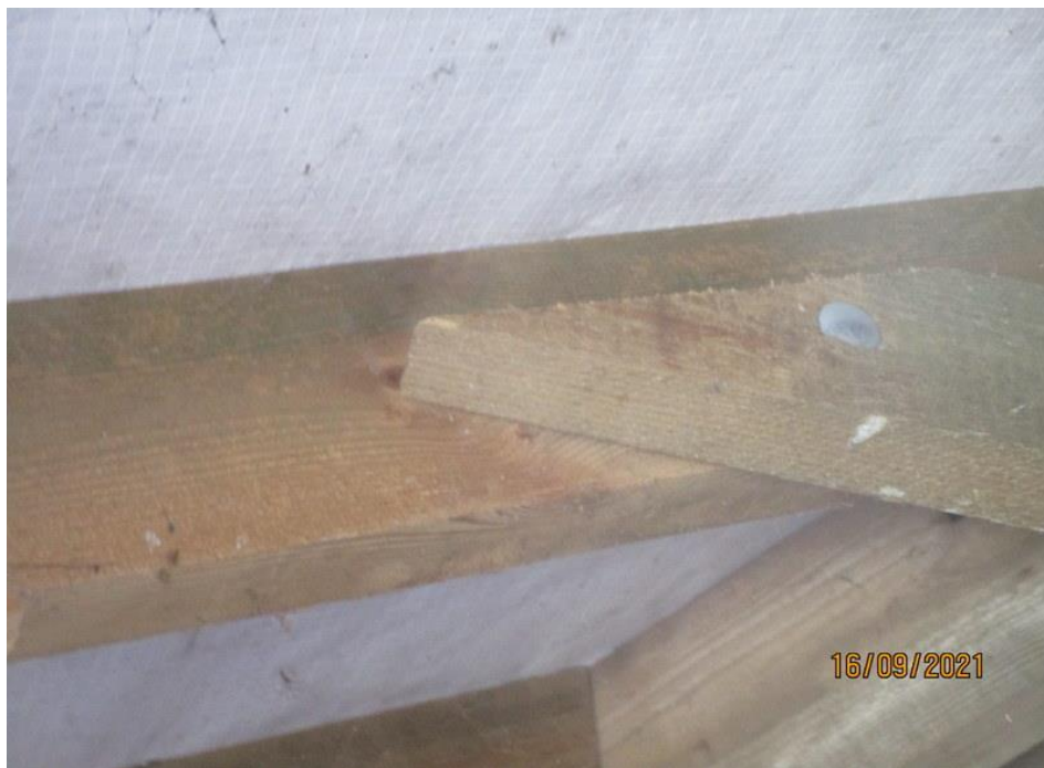
Roof timbers to the rear extension and underlay beneath the slates.
