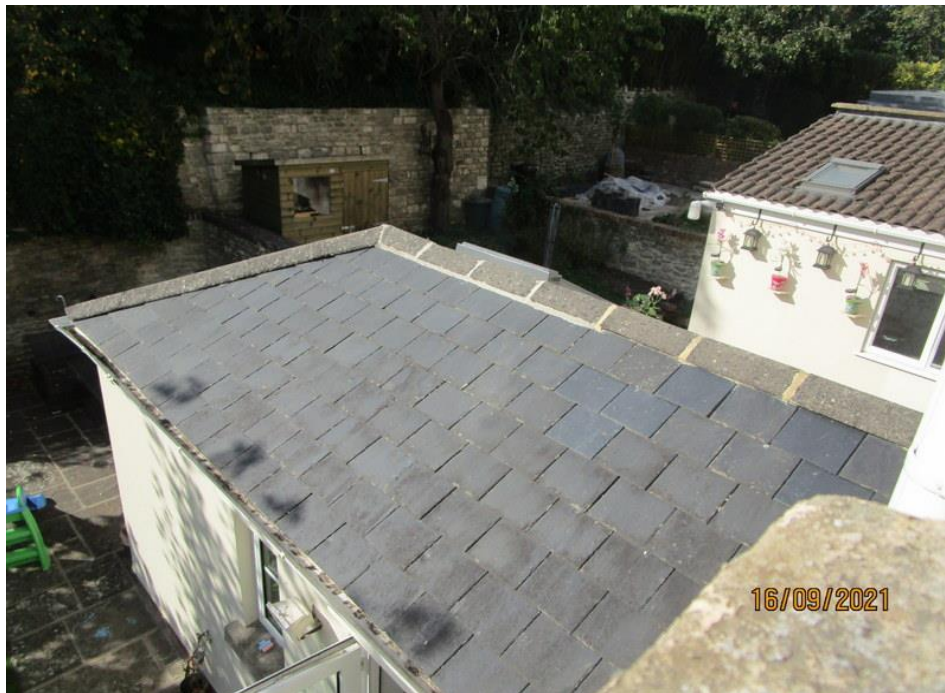
Slate roof coverings to the rear extension.
