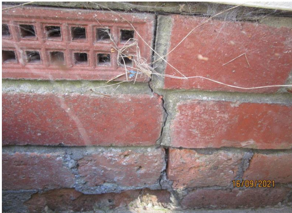
Cracking affecting the brickwork above ground level to the left rear.
