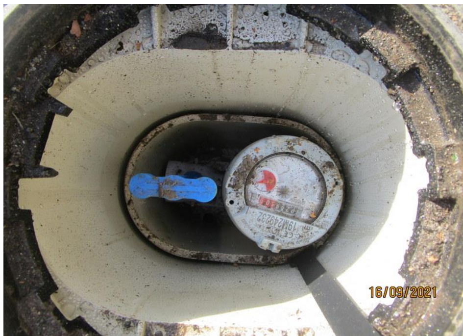
External stop-tap and water meter to the left side.
