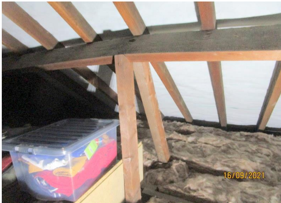
Rafters and purlin to the left side of the main property. Note distortion affecting the purlin timber above the strut.
