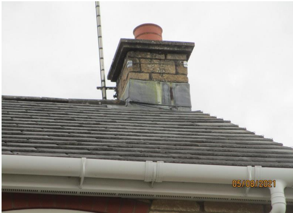
Chimney and roof coverings viewed from the front showing also plastic rainwater fittings.
