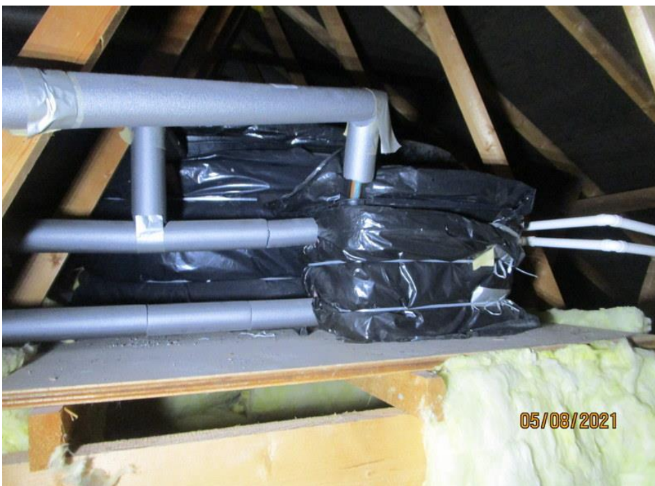
Cold water tanks in the loft.
