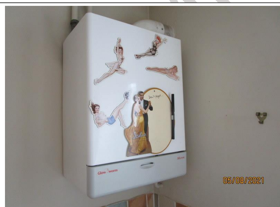
The gas central heating boiler located in the kitchen.
