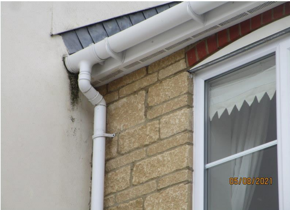
Signs of overspill around the downpipe to the right rear of the property.
